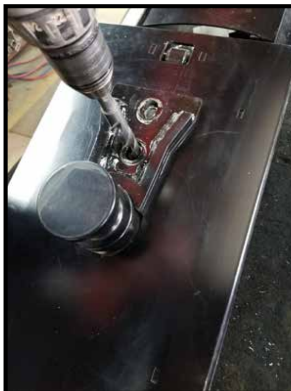
3. Drill the marked holes with a 5/8" drill bit.
