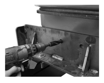
**3.** Center punch the drilled hole location and use a 29/32" drill bit to drill holes. Be sure to check for hose clearance on reverse side before drilling.
