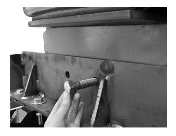
**4.** Install 7/8" x 3.00" bolts and nylon lock nuts into drilled holes and tighten to specified torque.
