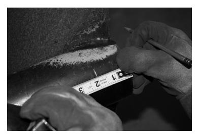
5. Drill 25/32" Hole through both walls of core tube 2" from end.
